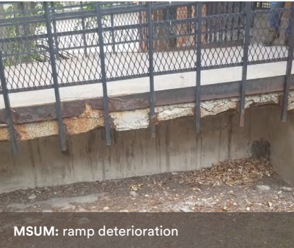
MSUM: concrete deterioration
